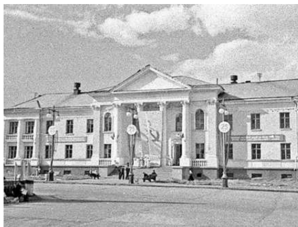
Figure 8: Completed Children's Hospital building in Vorkuta, 1950 (Vorkuta pokazhet Sever, N.D.)
