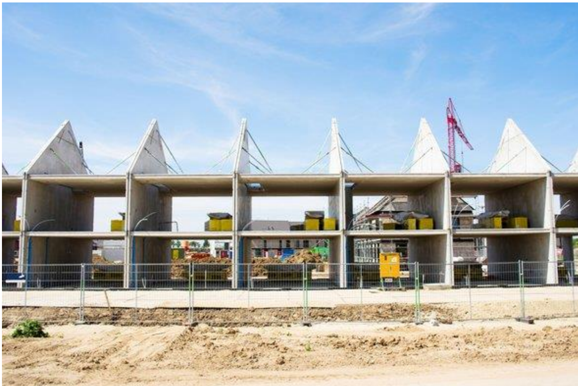
‘Terraced houses under construction in Nijmegen, Netherlands’ door Marcel Rommens (bron: Shutterstock )
