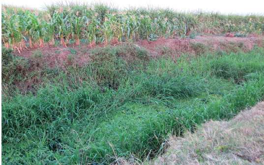
(c) Drainage canal with aquatic weeds
