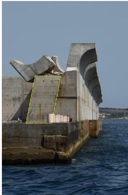
**Figure 1.** Civitavecchia’s crownwall failure. Yellow dashed line highlights the additional concrete wall that was constructed on a later stage.
