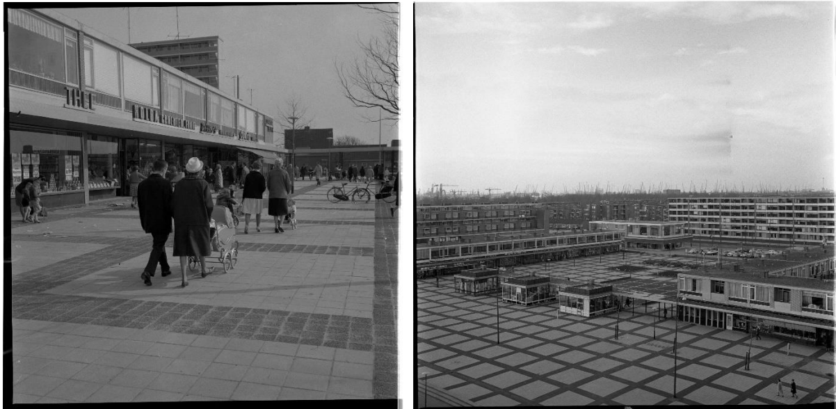
Figure 23, Images of Plein 1953 shortly after its completion. Source: Stadsarchief Rotterdam
