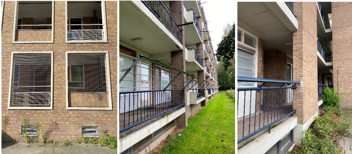
Figure 10, extra barriers on the ground floor to create a sense of security
