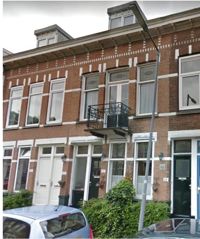
Street view of the building (Huispedia, n.d.)
