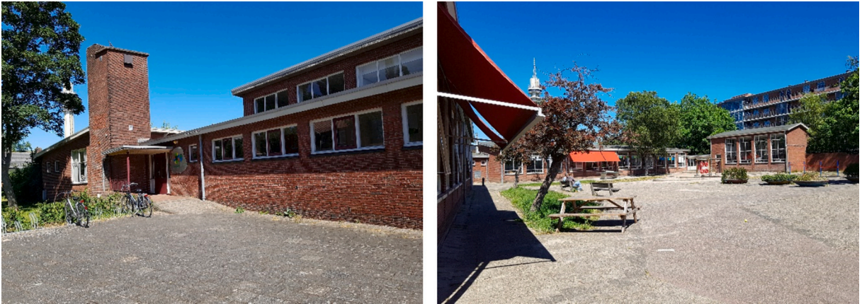
Fig. 2. Photos of the existing school building in the original state.
