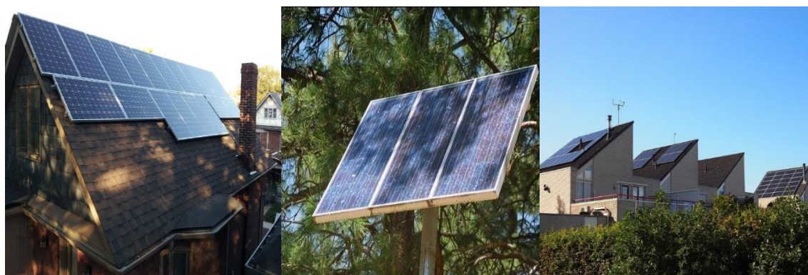
Figure 1.2: Solar panels under partial shading conditions
