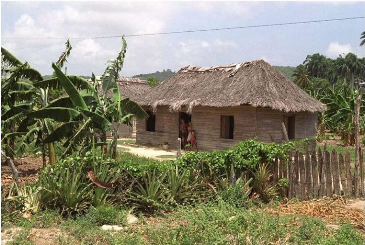
Figure 6: Bohío built with wooden boards. The Spanish settlers started modifying the traditional Taíno homes by adding windows and doors. Retrieved from: Soraluce, J.R. (2003). El Bohío Cubano, Arquitecturas de Cubierta Vegetal en el Caribe. El Pajar. Cuaderno de Etnografía Canaria. II Época (de A Coruna), p. 144-147
