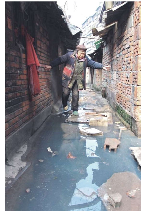
Aging drainage system.
