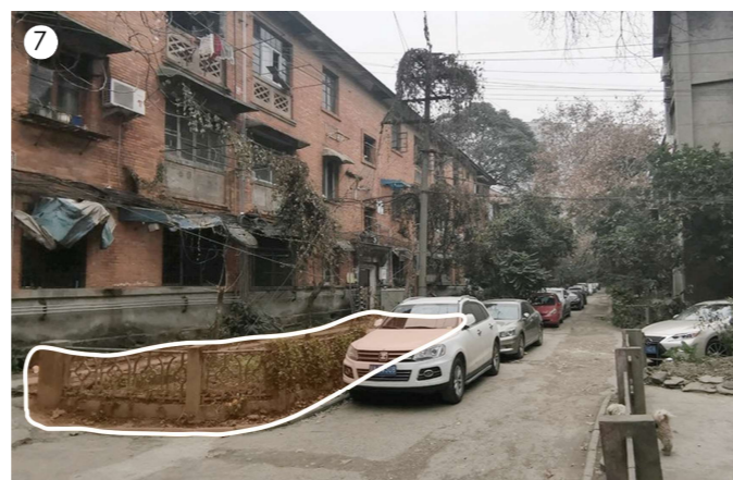
7 The green space at the front of the building separates the building from the road and protects the privacy of the residents. However, the green space has only some grass cover, is fenced off and is not fully utilised.
