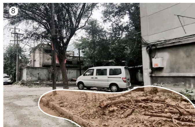
8 The green space to the side of the building has been left untended and is derelict
