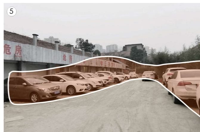
5 Due to the construction of the subway station, the building in front of the station area was demolished and is currently used as a parking lot.
