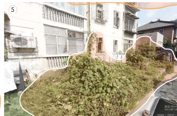
5 The hard paving on the sunny side in front of the building has been transformed into a vegetable garden by the ground floor residents by laying down soil.
