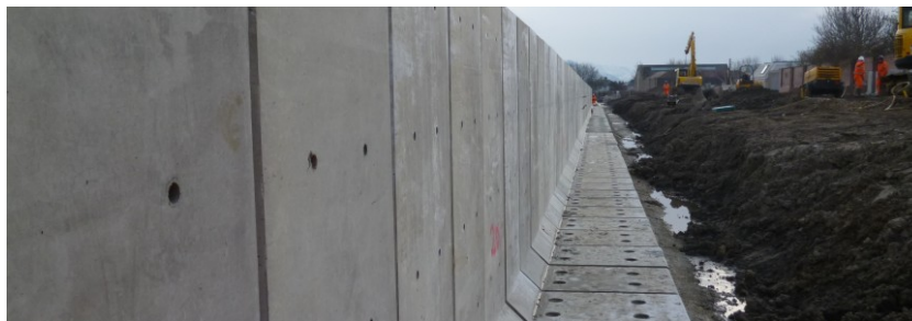
Figure 2.18: A simple L-shaped retaining wall. Photo by Marshalls CPM.
