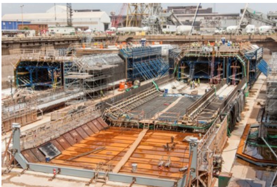
(a) Construction of the tunnel element. Photo by Doka.
