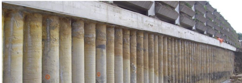
Figure 2.16: Concrete pile wall with heavy top load. Photo by Geotech Rijeka.
