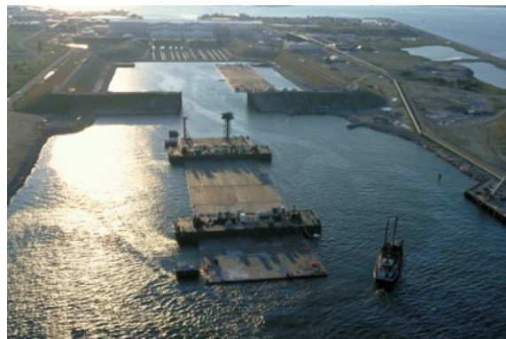
(b) Transportation of the tunnel element. Photo by DIMCO.
