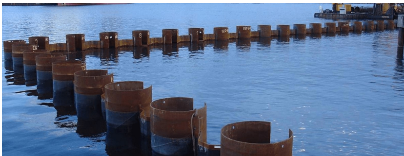
Figure 2.15: Example of a combi wall in water. Photo by Oriental Steel Pipe.
