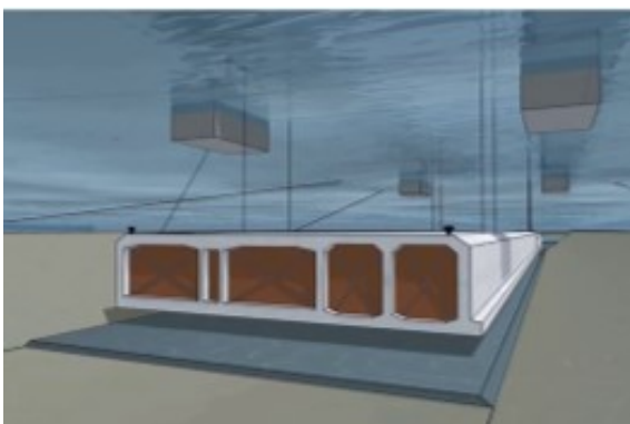
(c) Immersion of the tunnel element. Image by RambolGroup.
