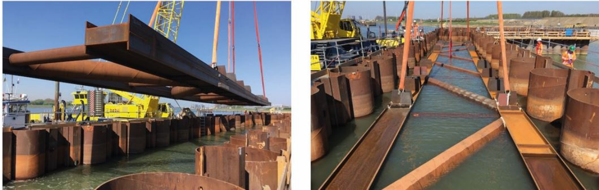
Figure 3.9: Construction of the end wall including framework. Photos by BAAK.
