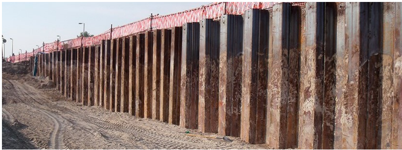
Figure 2.14: Example of sheet piling. Photo by Swissboring.
