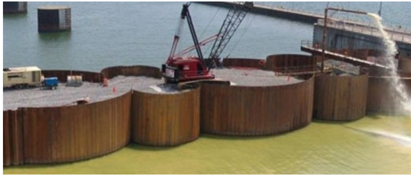
Figure 2.20: Cellular cofferdam. Photo by C.J. Mahan Construction Company.
