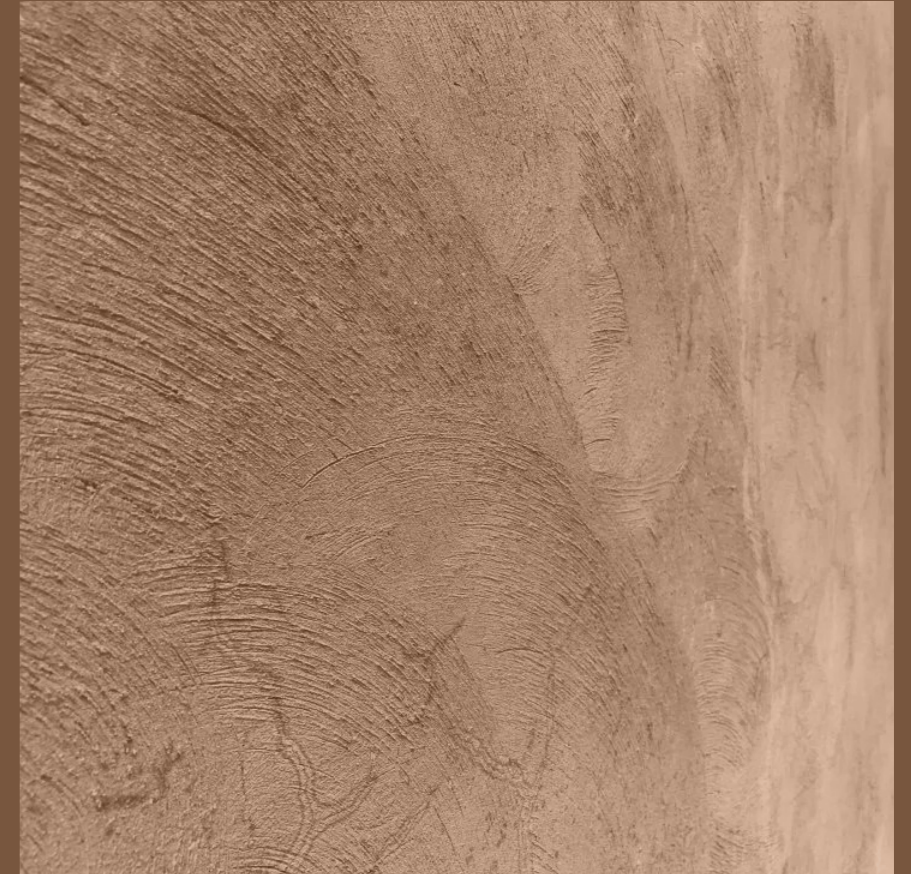
Cement plaster Finish
