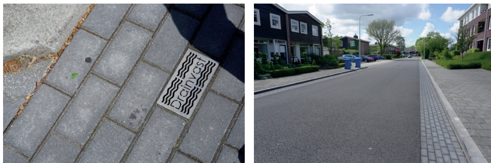
Figure 4-6. Case #33 has been assigned the root cause incomplete knowledge about the internal technical processes. The pavers were separated by joints filled with a permeable material, allowing water to infiltrate. Even after a small rainfall event, however, water remained ponding for at least one hour. As such, it was thought that the permeable material had become clogged, leading to a malfunction of the SUDS.
