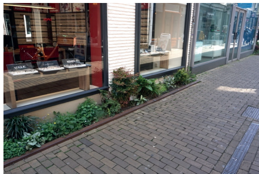
Figure 4-3. Case #30: a facade garden, which has been assigned the root cause embedded practices of involved actors. A facade garden is typically constructed surrounded by raised borders. Preventing runoff to be drained into the garden, this reduces the effectiveness of the SUDS.
