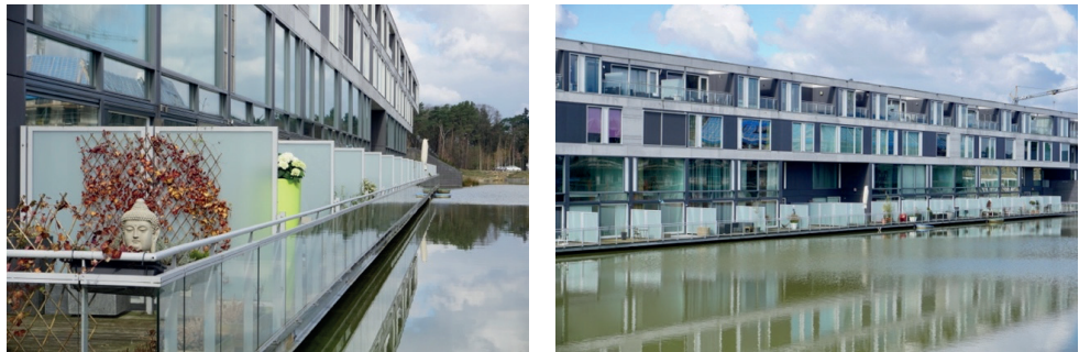
Figure 4-4. Case #60 has been assigned the root cause poor communication between different actors. Due to lacking communication between the architect and the municipality, the houses were built only 0.15 meter from the water level. This minimized the storage capacity of the surface water, while the water was initially designed as a storm water detention pond with a freeboard of 0.70 meter.
