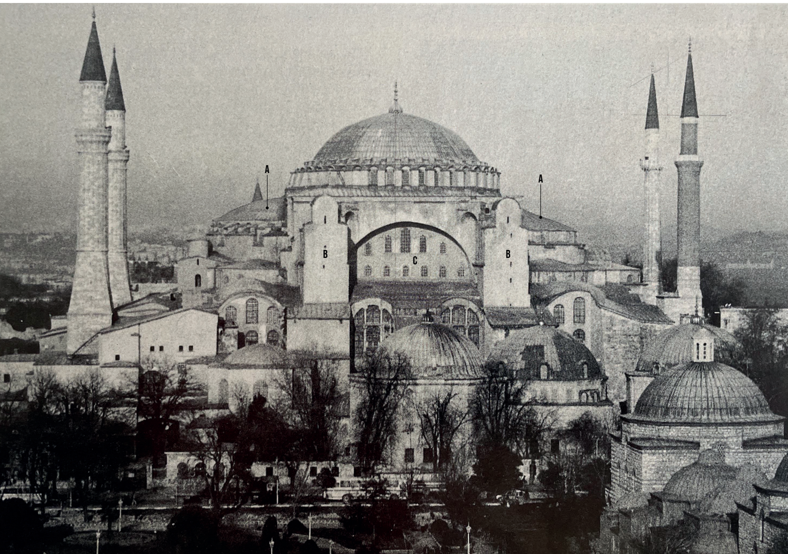
Figure 1.2 The church from the south (Hagia Sophia: Architecture, Structure and Liturgy of Justinian's Great Church 23 - R. Mainstone)
