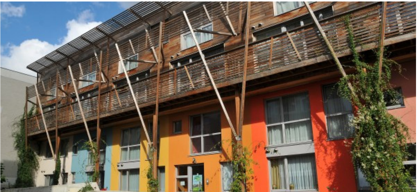
Figure 8: Housing projects L'écluse by CLT Brussels.
