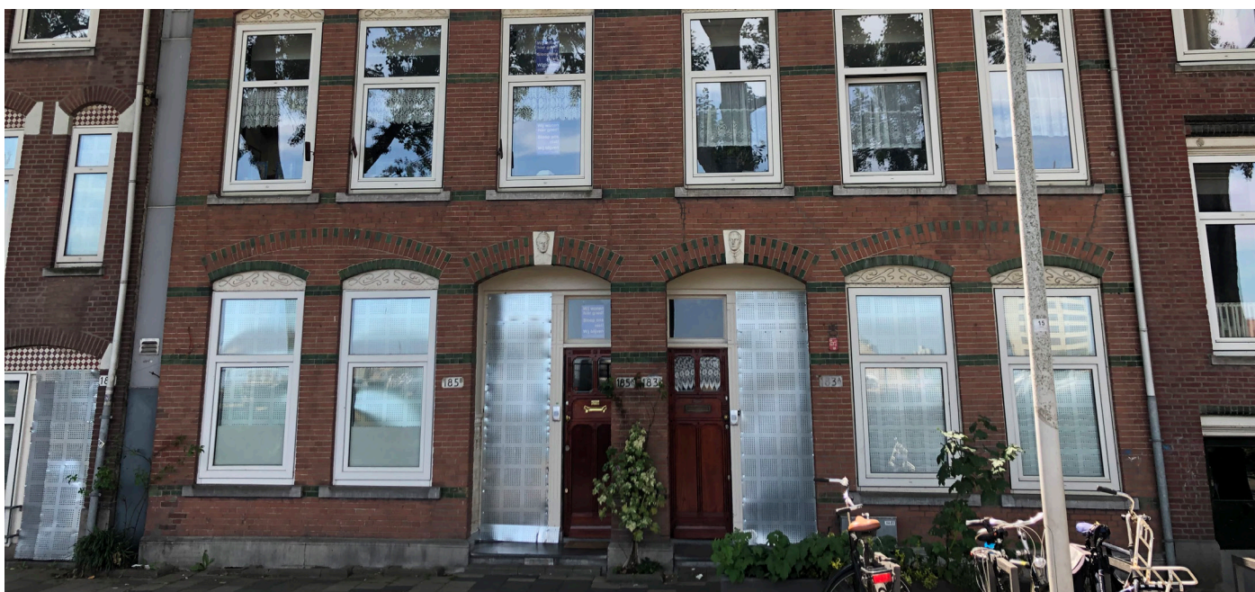
Figure 21: Some of the blocks eligible for demolition in De la Reystraat (top) and Hilledijk (bottom). Many have already been shuttered to prevent squatting.
