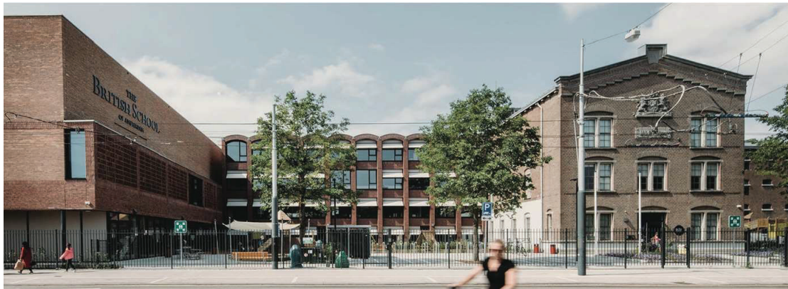
Figure 2. The British School of Amsterdam after the transformation. Source photos atelier PRO architects, photos by Eva Bloem
