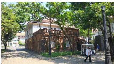
(a) west facade of the building.
