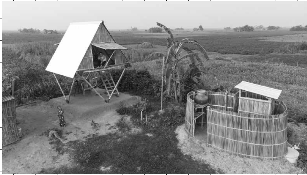
Photograph of a housing system of mobile modular structures made from bamboo; Khudi Bari. Photographed by Asif Salman.
