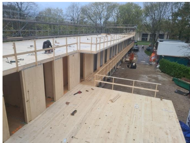
Figure 8: Left: Diagram of Grote Kreek structure showing CLT walls and floors. Right: Photo of the building under construction. Retrieved from https://www.ucarchitects.com/projects2/grotekreek/# on 8-11-2022.
