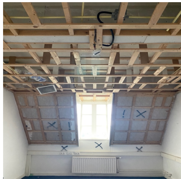
Figure 11. A room prepared for selective demolition
