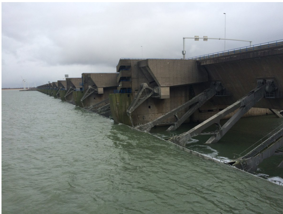
Figure 1.3: Highwater at the Haringvliet Sluice complex (December 8th, 2017), from Rijkswaterstaat (2017b).
