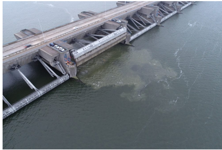
Figure I.3: Plungeline during current Kierbesluit clearly visible from an aerial photo, photo from Rijkswaterstaat.
