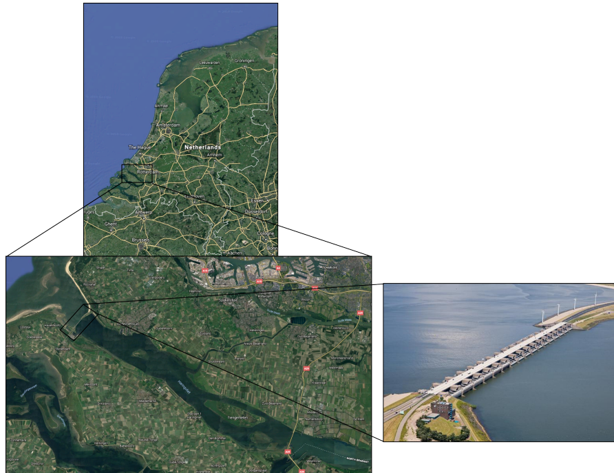
Figure 1.1: Location of the Haringvliet (Google Earth, 2018) and an overview picture of the Haringvliet sluice complex (Interprojectmanagement, 2015).
