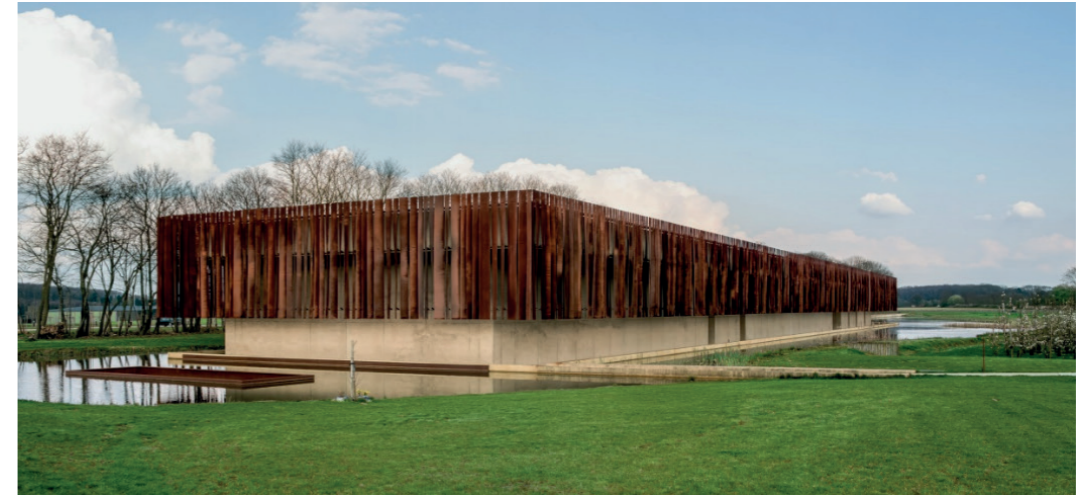
Figure 5.026 – Hofheide crematorium, RCR architects (2015) • Source: El Croquis
