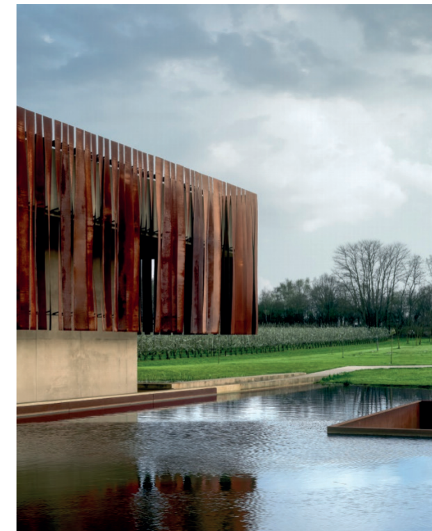
Figure 5.027 – Steel skin, Hofheide crematorium, RCR architects (2015) • Source: El Croquis
