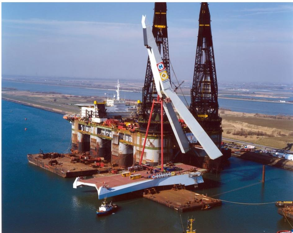
**Figure 1.2:** The installation of the pylon of the Erasmusbridge by Heerema MC's SSCV Thialf in 1995
