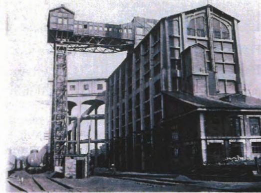
Figure 30: Reinforced concrete construction of the Blast furnace of the Coke-chemical plant in Tscheglovo (Kemerovo), designed by Olivier Piëtte, 1916.
