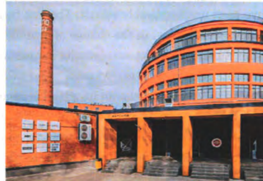
Figure 4: The Bread factory number 9 in Moscow after the transformation to the department store 'Marsakov', 2019.
