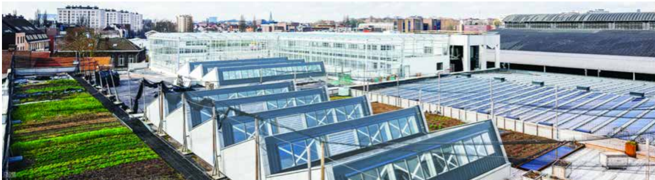
Figure 32: The Ferme Abbatoir's Building Integrated GreenHouse (BIGH) in Brussels is one of the prime examples for value-added benefits and entrepreneurial partnership. Images courtesy of BIGH.
