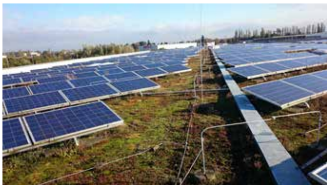
Figure 18: Being Beneficial with Big Healthy Footprints. Water retention via thin-layer extensive roof on retailer building. Image NIRA GmbH & Co. KG.
