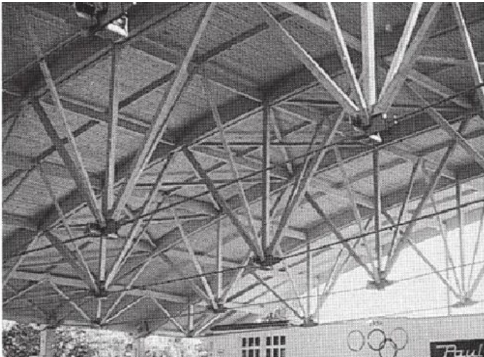
87. Fish belly truss with steel tie
