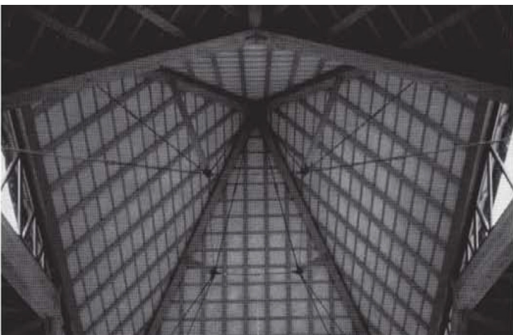
85. hip roof with tensility
