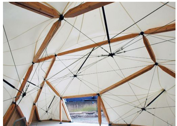
Figure 18, timber frame structure with fiber skin
