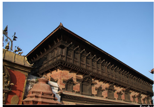
Figure 31. crossing frame non-structure element
