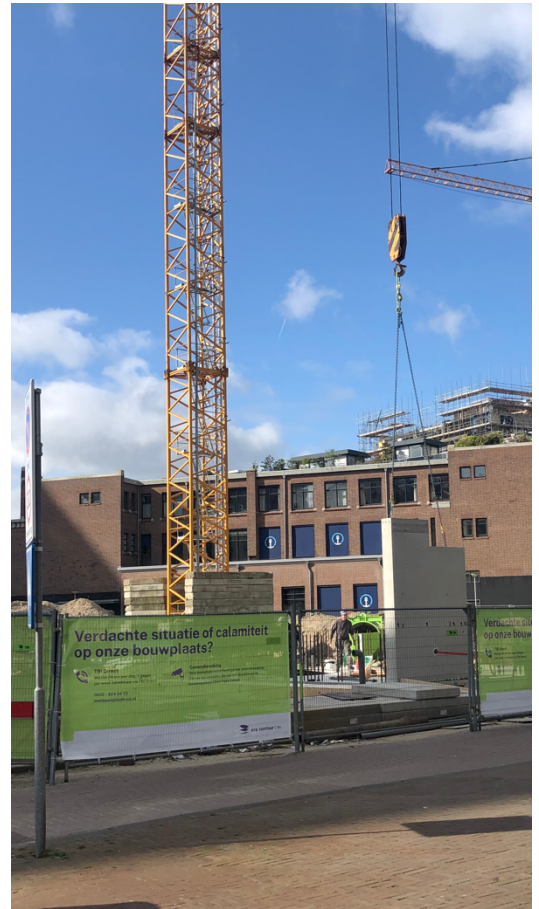
Image 5. Construction process – Sawa.
