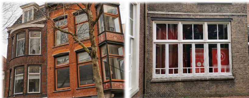
Fig. 1. Unreinforced masonry walls with large openings in the Netherlands.
