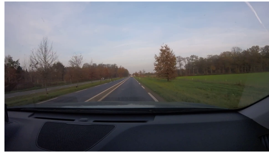
Figure 3.6: View front camera
