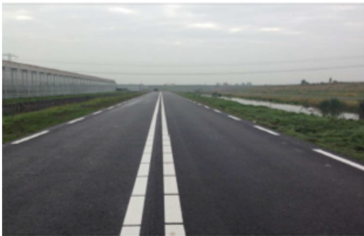
Fig. 1. Type 1 lane marking (paint or tape)
