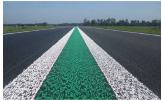
Figure 2.7: Application type 2 (dots or drops, profiled)
