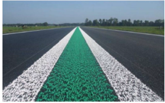
Fig. 2. Type 2 lane marking (dots or drops, profiled)
