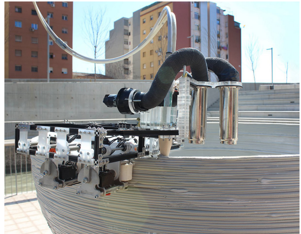
Figure 67. Prototype of a lunar habitat build with lunar regolith simulant using CC (Khoshnevis, et al., 2005).
