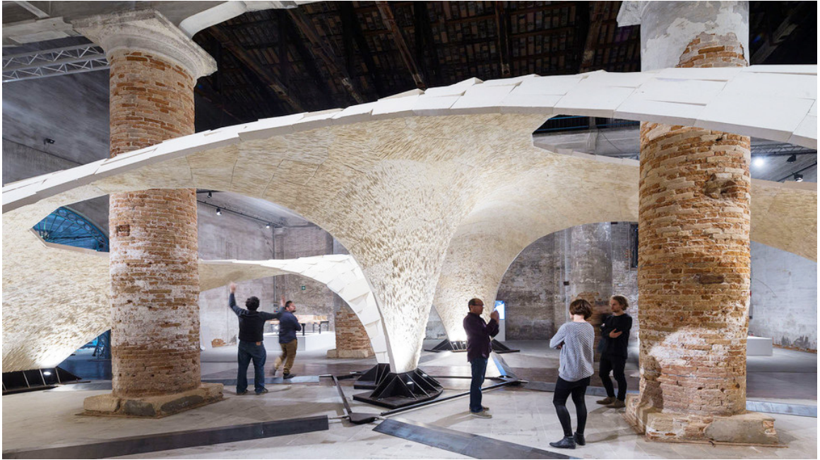
Figure 82. The Armadillo Vault for the Venice Biennale 2016. It comprises of 399 limestone panels with a minimum thickness of 5 cm spanning 16 m (Block Research Group, 2017).
