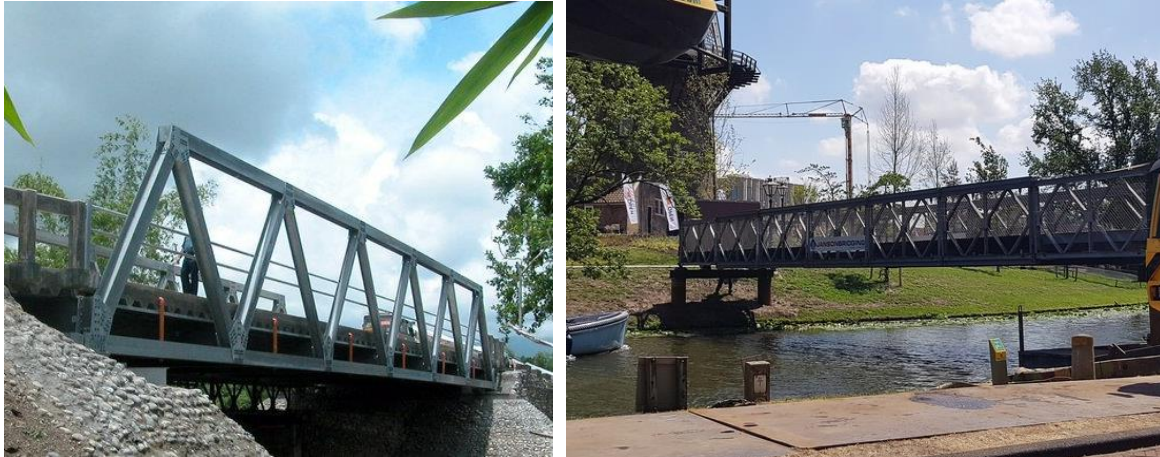
Figure 5: Waagner-Biro modular steel truss bridge (left) (Waagner-Biro, 2012) and temporary Janson bridging structure (De Waard, 2018)
