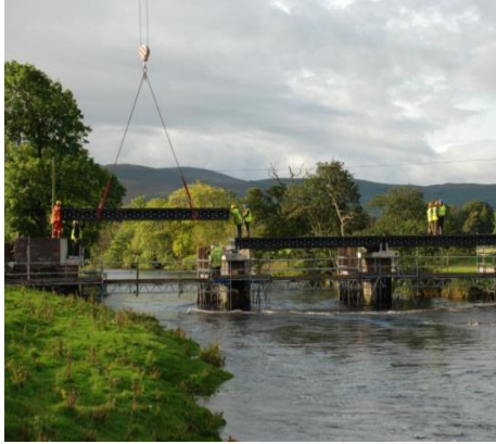
Figure 4: Assembly of the integrated deck girders of the bridge onto the supports (left) and a cross-section of the bridge (right) (Kim, 2011)
