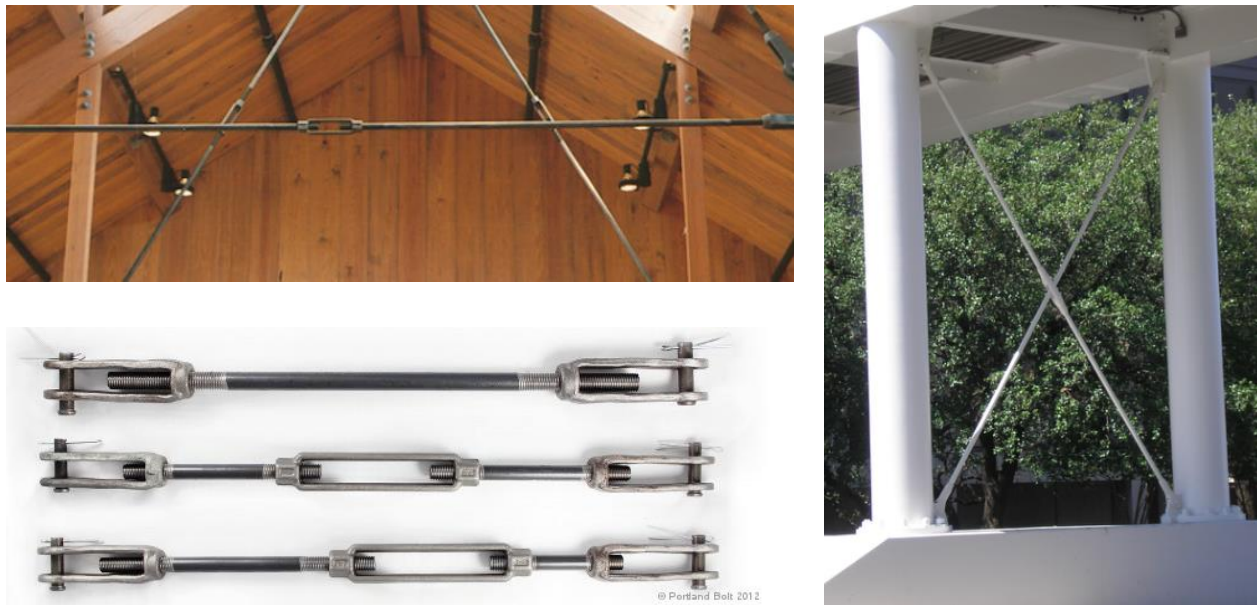
Figure 45: Various examples of uses of tied rod constructions with turnbuckles: timber roof structure (top left) (Architectural Timber & Millwork, Inc.), close-up of turnbuckles and threaded rods (bottom left) (Portland Bolt), stability bracing for a walkway (right) (HALFEN)
