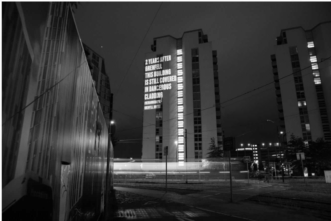
"2 years after Grenfell this building is still covered in dangerous cladding."/ 2019
