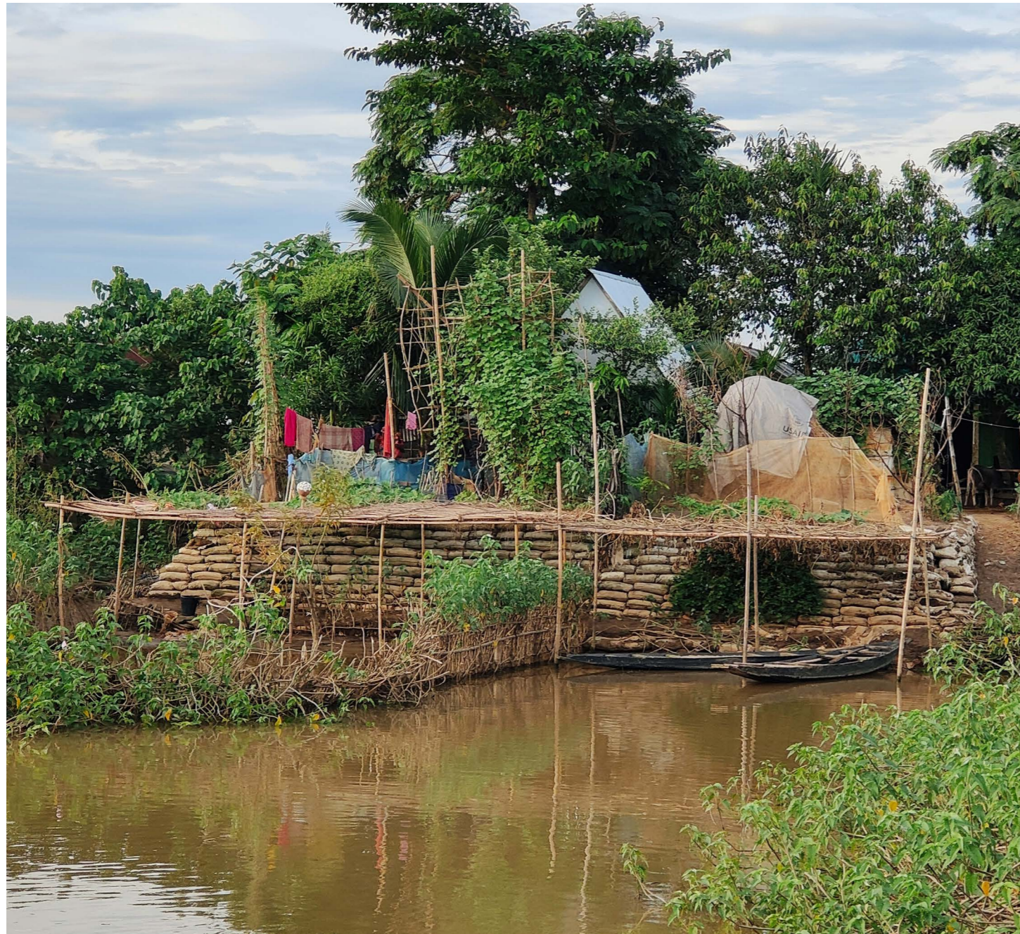
Figure 7. Housing in haor in Tahirpur. Author own photograph
