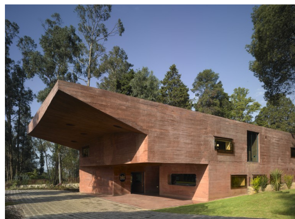
Figure 25: Entrance of the chancellery, seen from the northeast. Cantilever providing shade on the east end of the building. From "Embassy Ethiopia / Bjarne Mastenbroek and Dick van Gameren," by Archdaily., n.d. ( https://www.archdaily.com/198254/embassy-ethiopia-bjarne-mastenbroek-and-dick-van-gameren/5004d8b928ba0d4e8d0007ed-embassy-ethiopia-bjarne-mastenbroek-and-dick-van-gameren-photo ).
