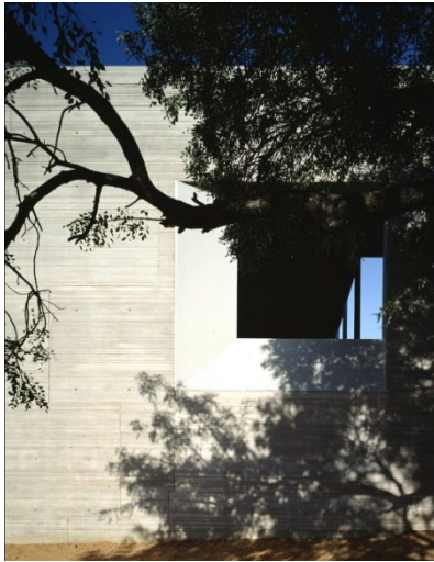
Figure 12. The rock-like appearance from the concrete façade blends in with its surroundings. From "Netherlands Embassy Mozambique," by KAAAN Architecten, n.d. ( https://kaanarchitecten.com/project/netherlands-embassy-2/ )
