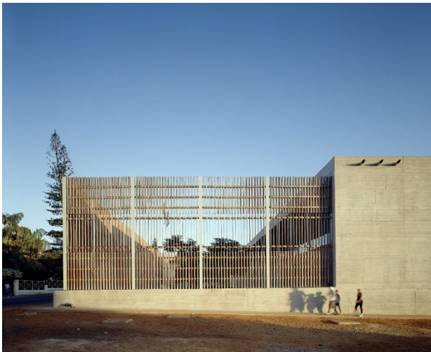
Figure 8. The high wooden fence around the inner garden with concrete base. From "Netherlands Embassy Mozambique," by KAAAN Architecten, n.d. ( https://kaanarchitecten.com/project/netherlands-embassy-2/ )
