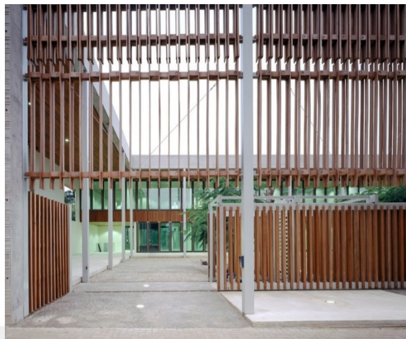
Figure 15. Open wooden fence, showing the transparent south façade. From "Netherlands Embassy Mozambique," by KAAAN Architecten, n.d. ( https://kaanarchitecten.com/project/netherlands-embassy-2/ )
