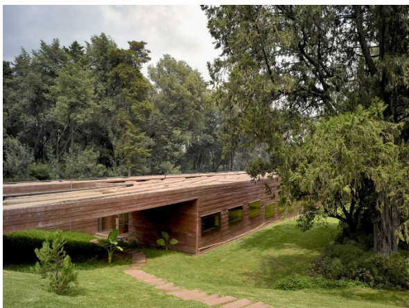
Figure 24: South façade with relatively small windows and canopy protecting from sun. From "Ethiopia Dutch Embassy," by Mecanoo., n.d. ( https://www.mecanoo.nl/Projects/project/72/Ethiopia-Dutch-Embassy ).
