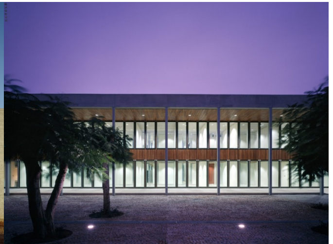
Figure 9. Steel veranda along the inner facade. From "Netherlands Embassy Mozambique," by KAAAN Architecten, n.d. ( https://kaanarchitecten.com/project/netherlands-embassy-2/ )
