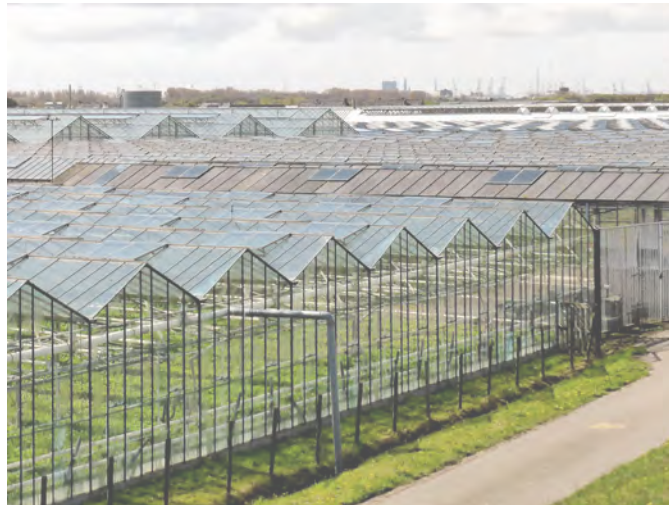
Fig. 19: Greenhouse structures in Westland. (Unsplash)
