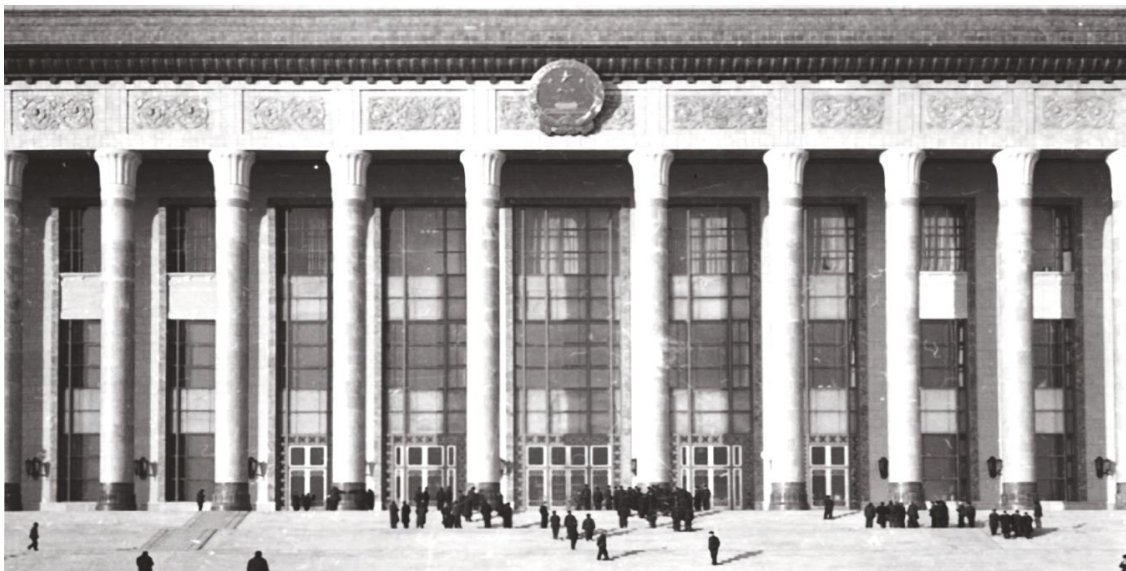
Fig 4-2 The mixed-style facade of the Great Hall with the distance between columns in the middle gradually increases
