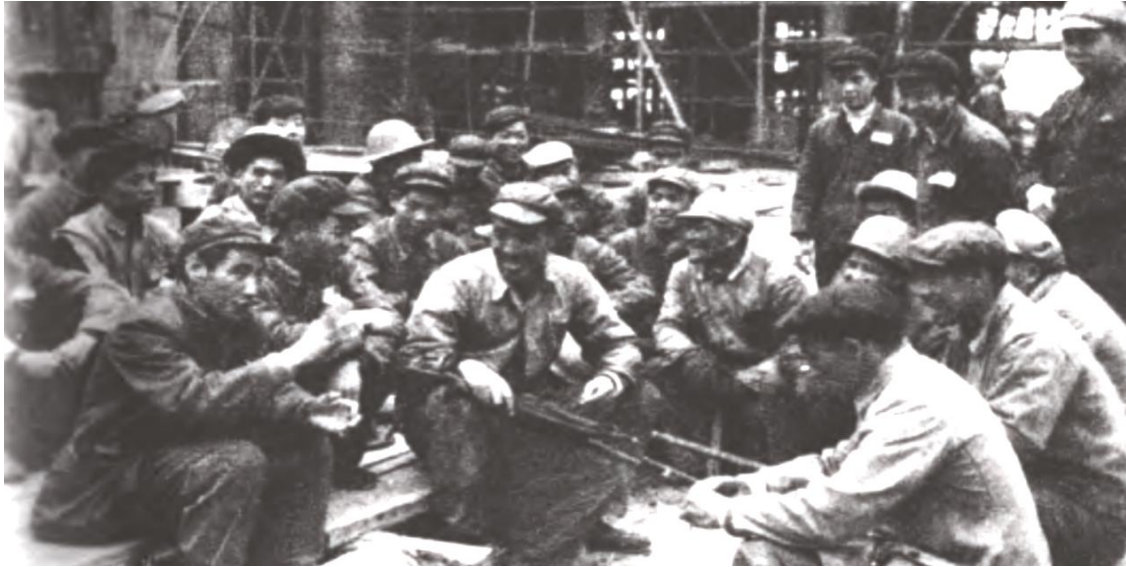
Fig 4-1 The discussion between officers, technicians and workers during the construction of the Great Hall
