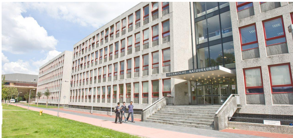
Figure 5. 3D model for Faculty of Applied Sciences (upper) and real picture of the entrance (bottom) (2016)
