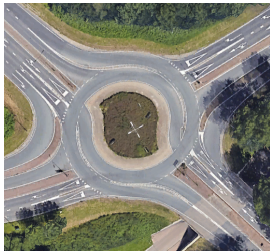
Figure 1.1: Aerial overview of a turbo-roundabout in Nieuwerkerk aan den IJssel, the Netherlands
