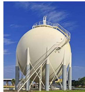
(b) Spherical pressure vessel
