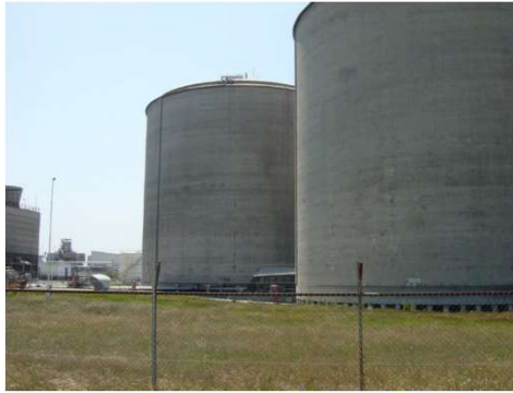
Figure 2.19: Refrigerated ammonia storage tanks at Europoort, Rotterdam
