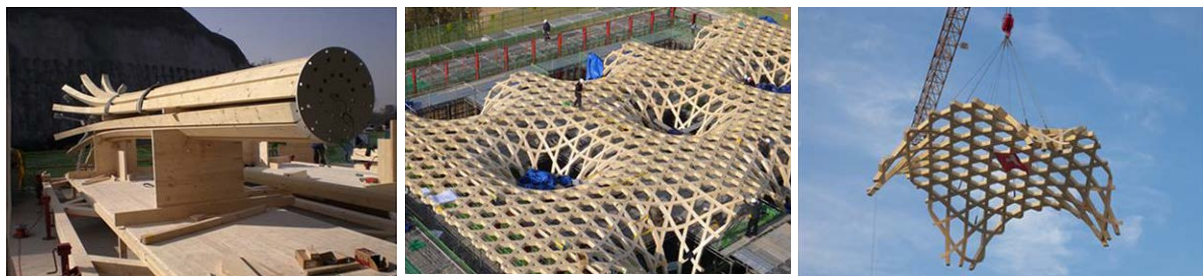
Figure 6. Hoisting construction process of Nine Bridges Country Club.
