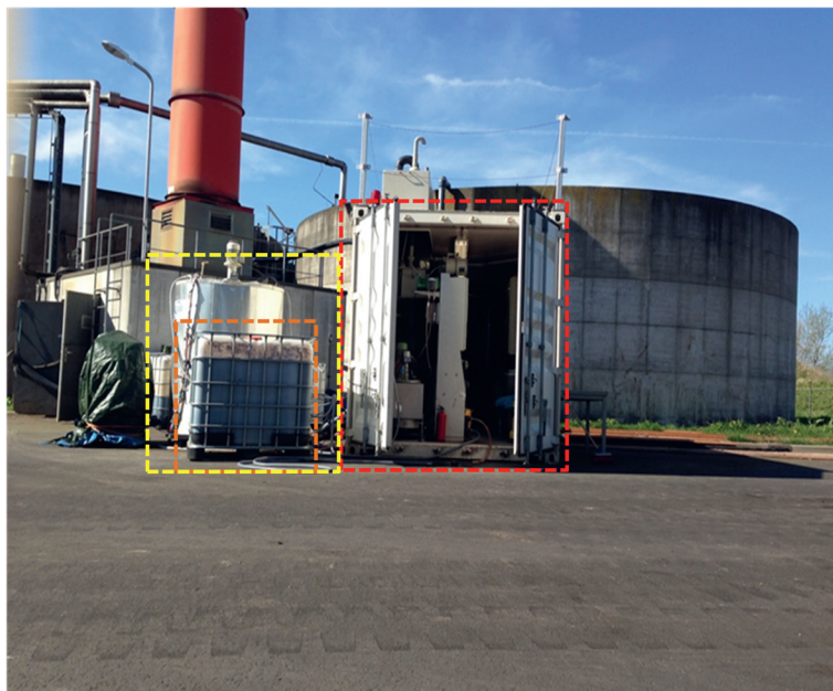
Figure 5.1 – Impression of the pilot plant. The open container contained the selector and accumulator bioreactor (red bracket). In the front, there is an IBC sedimentation tank (orange bracket). Behind the sedimentation tank, the influent buffer vessel was located (yellow bracket). (Image by Michel Mulders.)
