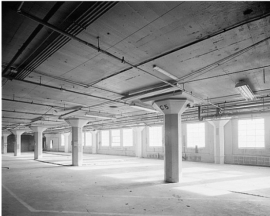
(a) Flat slab floor.
