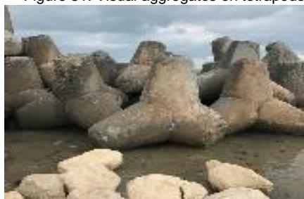
Figure 82: Broken tetrapod leg
