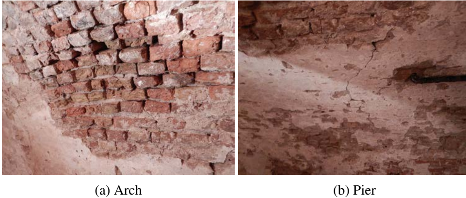
Figure 3: Investigation photos of the wharf cellar bond pattern.
