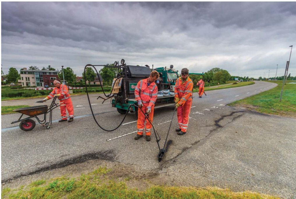
Figure 2-4: Filling cracks [32], image courtesy of CROW.
