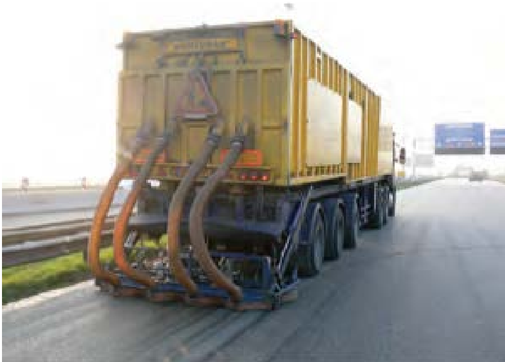
Figure 2-3: Focused water blasting. Image courtesy of Rijkswaterstaat.
