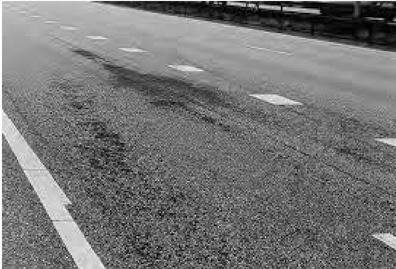
Figure 2-2: An example of raveling [58]. Image courtesy of Rijkswaterstaat.
