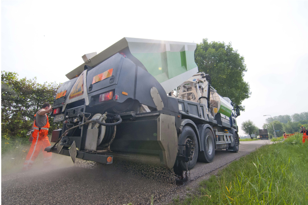
Figure 2-5: Surface treatment [23], image courtesy of Pavecare.
