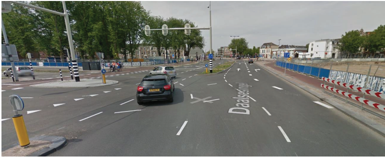
Figure 7.13: junction area with partial lane markings (source: Google)
