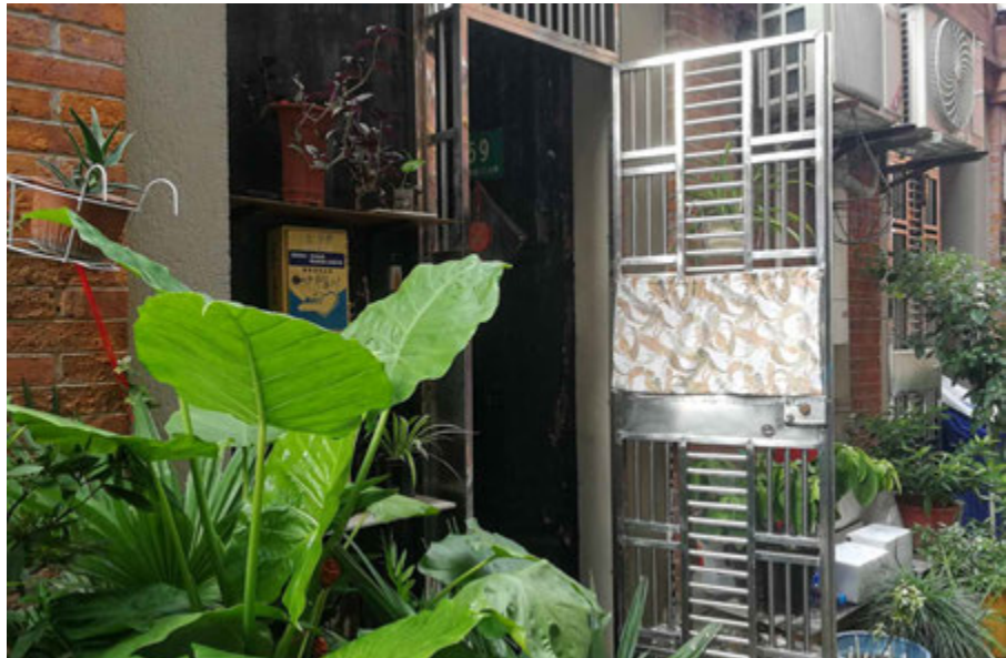
FIG. 8.24 The added stainless-steel anti-theft door on the outside of the original black timber gate of Bugaoli No. 59. Source: author, 2018.
