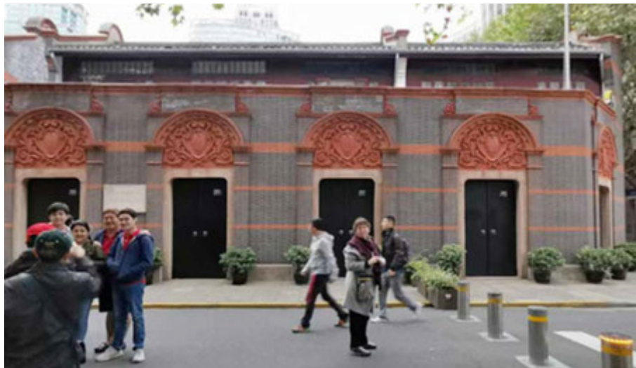
FIG. 6.11 Architectural façade of the Site of the First National Congress of the CPC, presented in an entirely new condition. Source: author, 2019.
