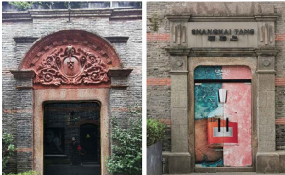
FIG. 6.9 Different curved stone or cement plastering pediments on architectural facades of buildings in Xintiandi after transformation. Source: author, 2021.
