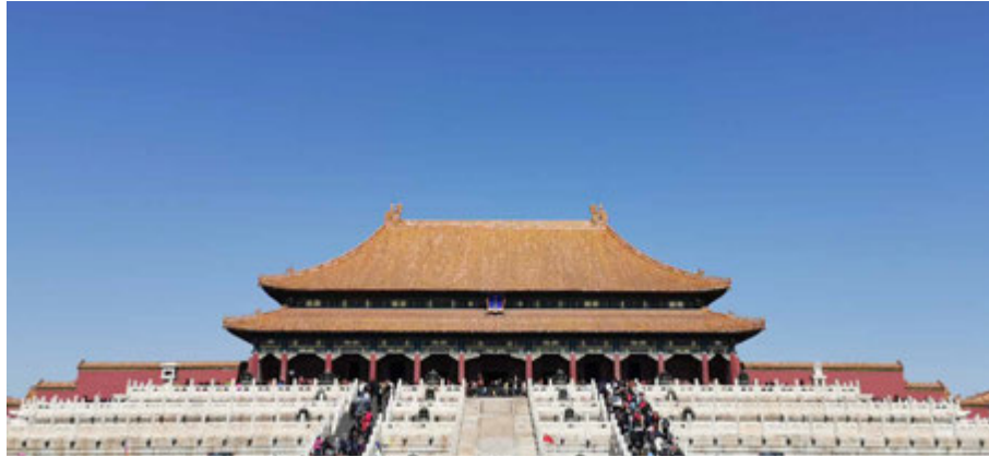
FIG. 3.5 The hip roof with double eaves is the highest form of roofing style in China's ancient architecture. This roof style is applied to Hall of Supreme Harmony (Taihe Dian, 太和殿), the largest hall in the Forbidden City, to reflect imperial power. Source: author, 2019.
