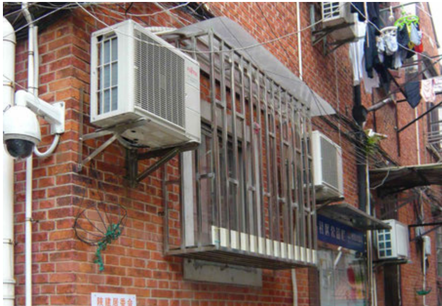
FIG. 8.23 The added stainless-steel window grilles and air conditioning mainframes on the façade of the historic building. Source: author, 2019.
