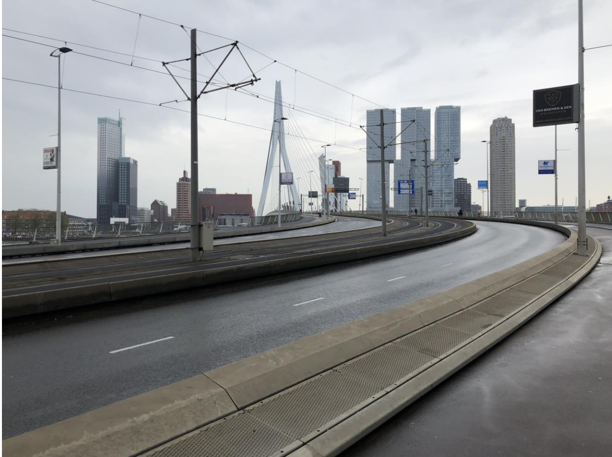
Deserted public space in Rotterdam, the Netherlands. Image by Maurice Hartevelde.
