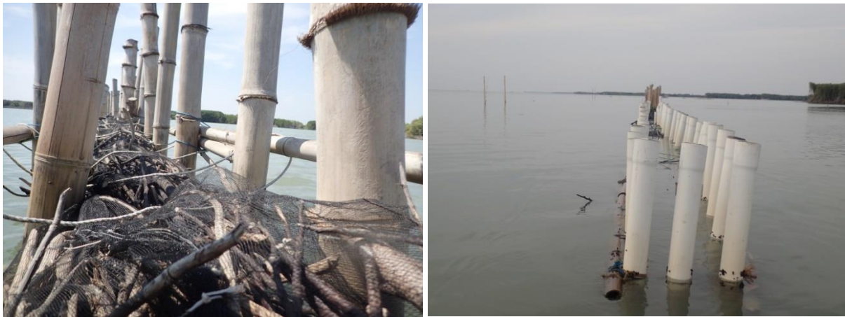
Figure 5.24 (a) Structure with brushwood fill material (Gijón Mancheño, 2017) (b) Structure without brushwood fill material (Gijón Mancheño, 2017)
