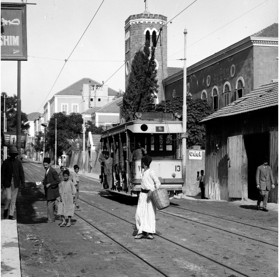
Figure 01: Electrified tram towards Ras Beirut, 1900s (image retrieved from Old Beirut)
